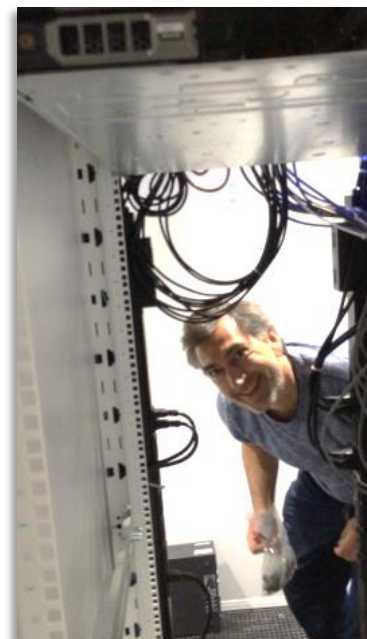
Tsvet & I Building "Rekall Cloud"
